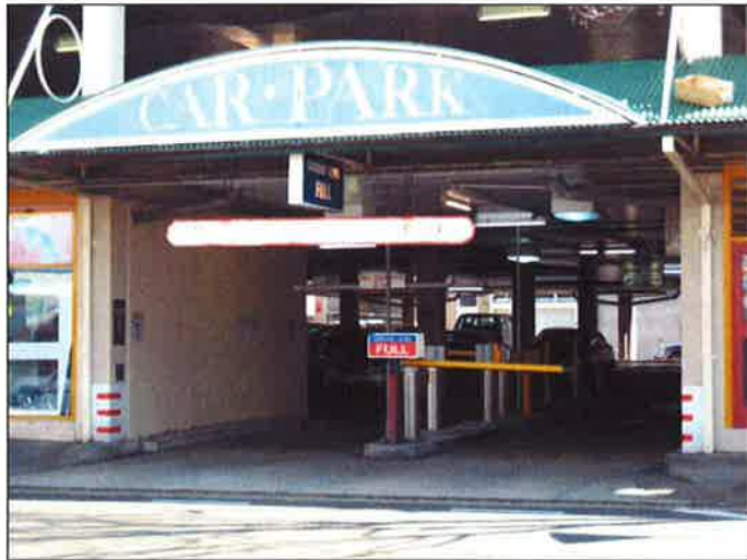
Photograph 5: View of existing entrance to Alexander Street car park ground level at Alexander Street frontage from eastern side of Alexander Street looking west.
