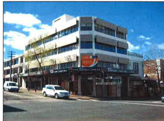
Photograph 13: View of existing 4 level office building opposite the site at the north-eastern corner of Alexander Street and Falcon Street.
