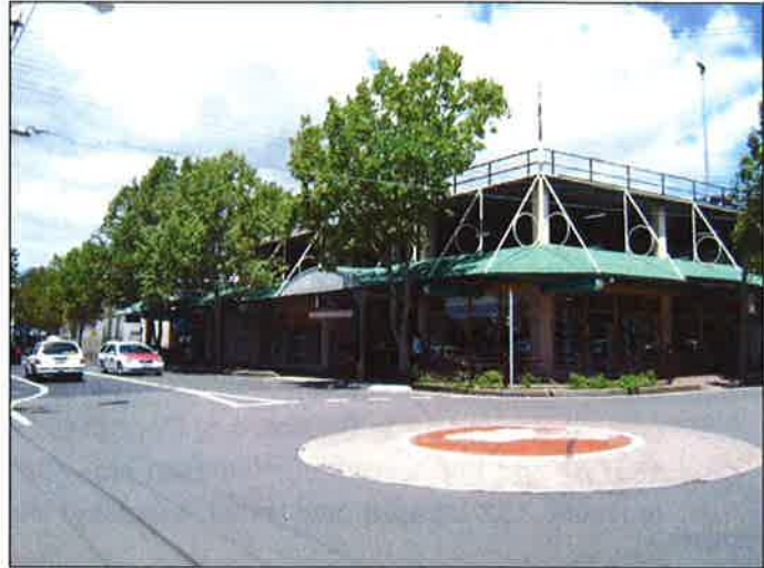
Photograph 1: View of existing car parking structure looking south along Alexander Street.
