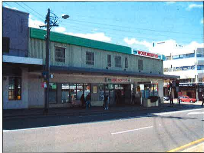
Photograph 7: View of Falcon Street frontage of existing Woolworths.
