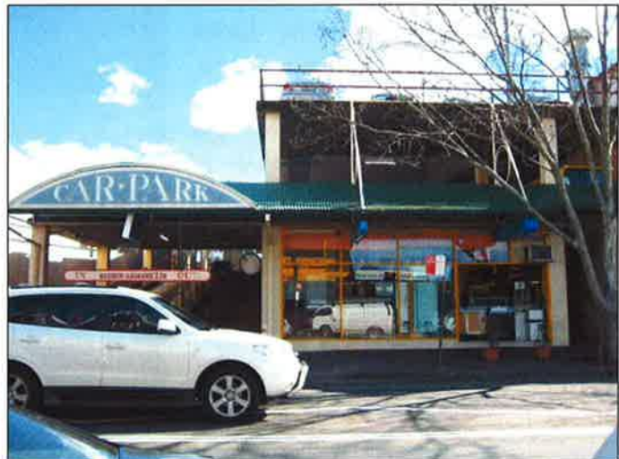
Photograph 4: View of existing entrance to Alexander Street car park levels 1 and 2 Woolworths located at Alexander Street frontage from eastern side of Alexander Street looking west.
