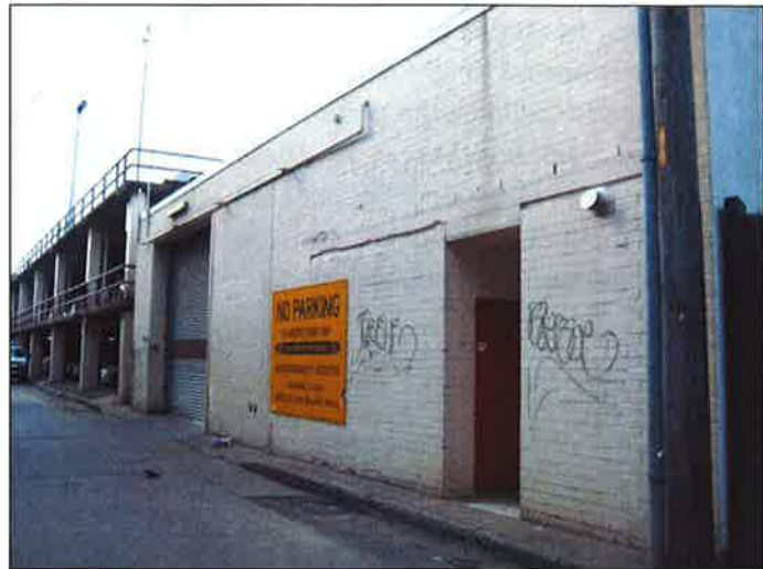
Photograph 9: View of Willoughby Lane frontage of the Woolworths loading dock and car park.
