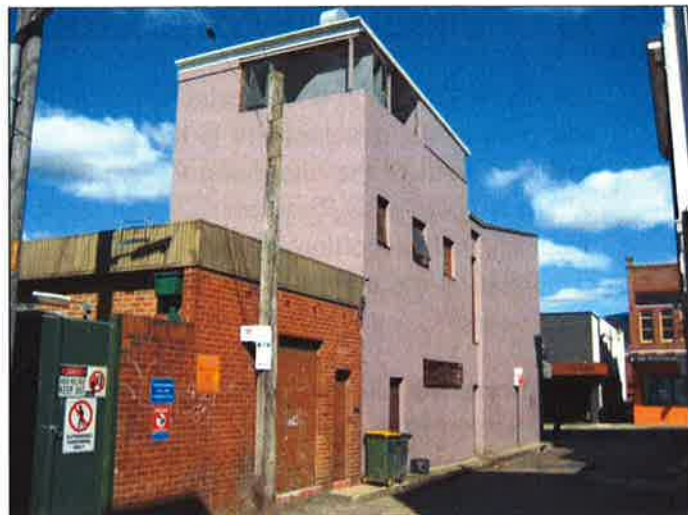
Photograph 8: View of Willoughby Lane frontage of the existing Energy Australia substation site.
