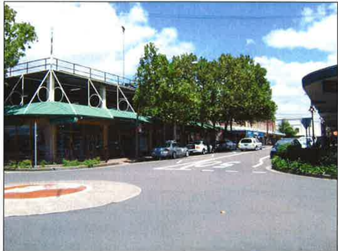
Photograph 2: View of the existing car park structure and shops looking west to the Burlington Street frontage.
